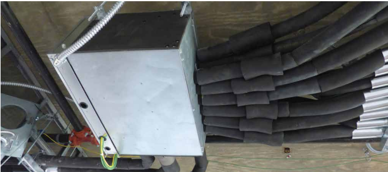
Insulation from Daikin Units to Branch Controller
